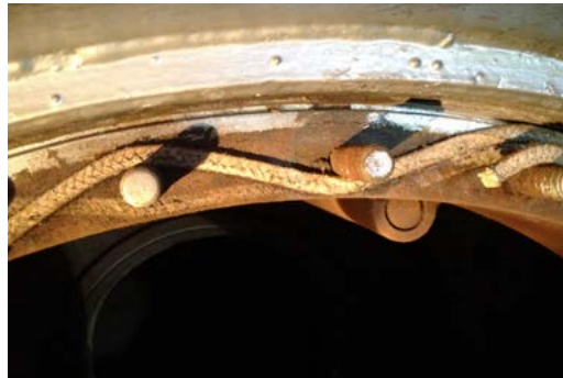
Joint tresse amianté
